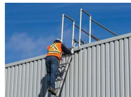
Hoops provide a solid grip and guardrails lead workers toward the center of the roof.
