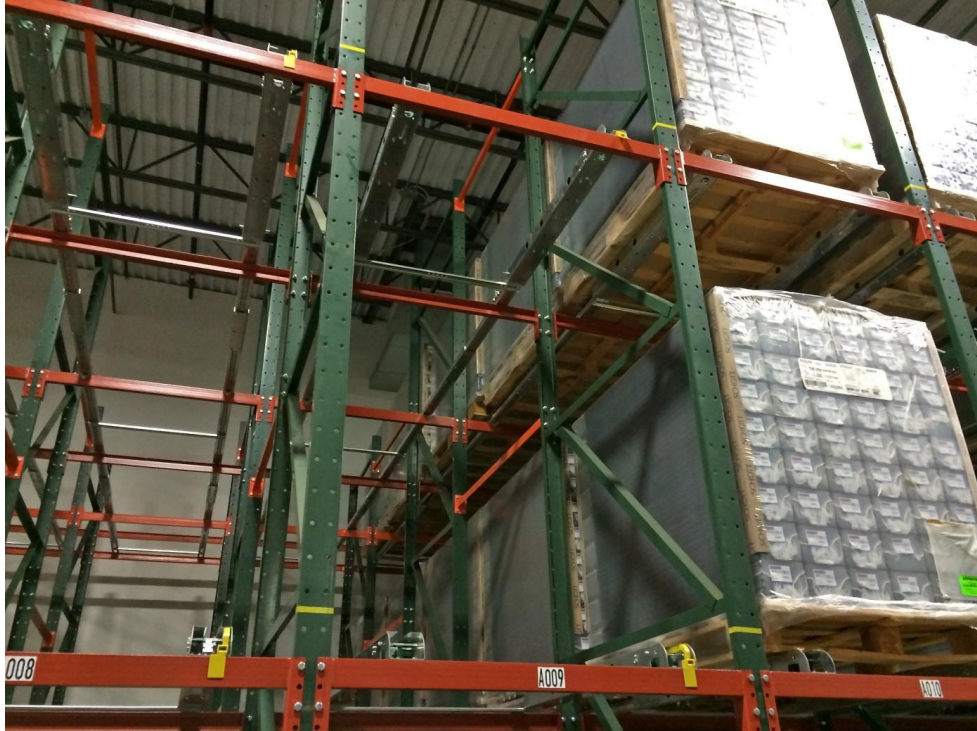
Drive-in retrofit: each storage lane can hold a different SKU
