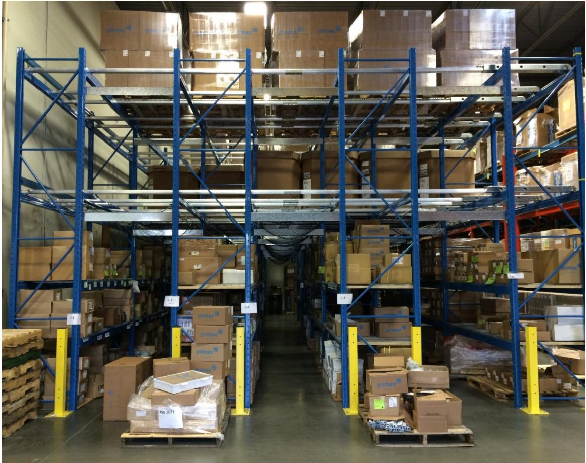
6 deep Flow-Rail above, picking aisles below
